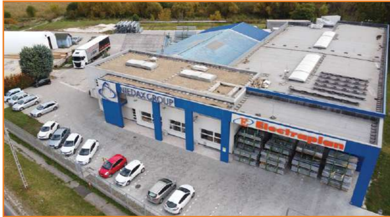
Headquarter in Érd
