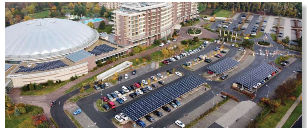
Budapest, Aquaworld - 400 kWp
