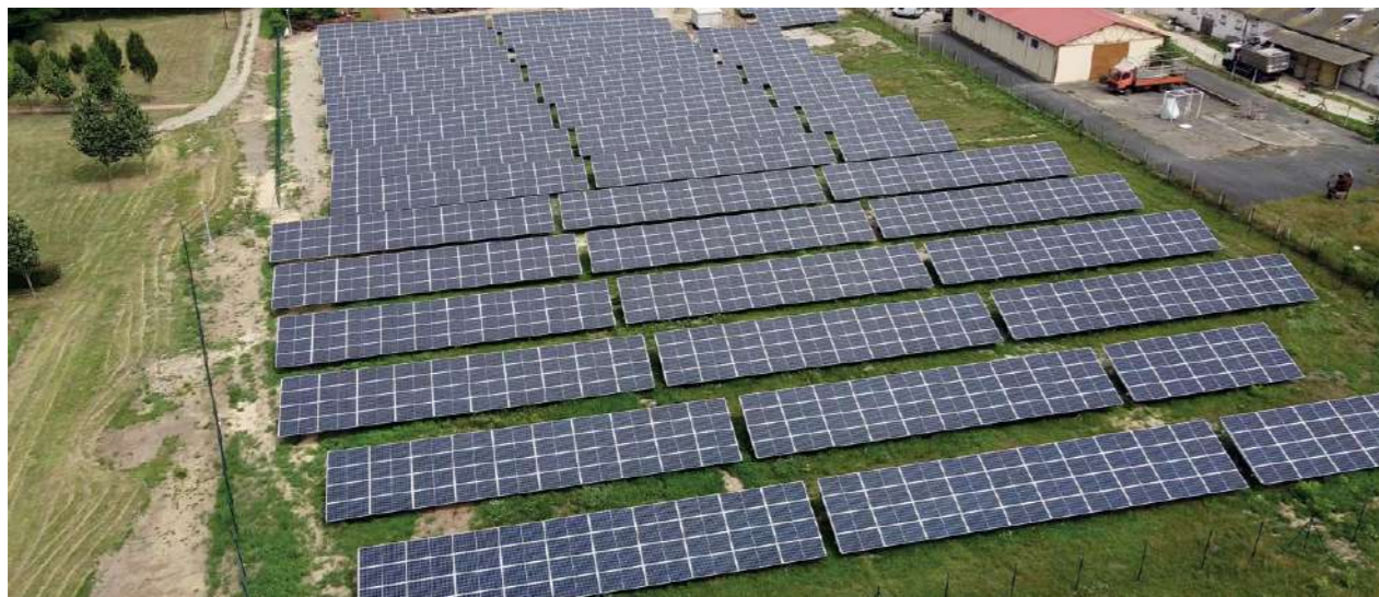
Óhid (Own power plant) - 500 kWp
